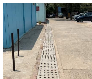
Rainwater Harvesting Drain
