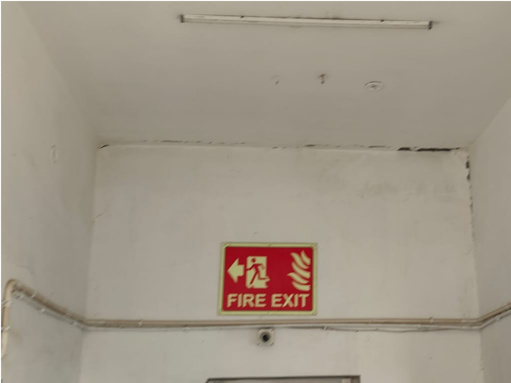
Crack at junction of building 2 & 3
