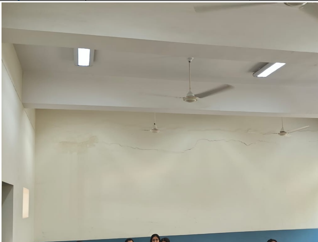
Horizontal Crack at the junction of Building 1 & 2
