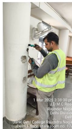
Photo 49: Half cell Potential Test is in Progress
