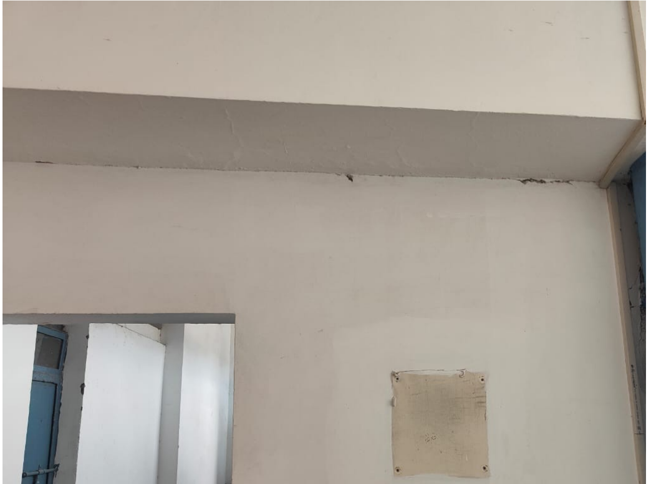
Crack at Junction of Building 2 & 3
